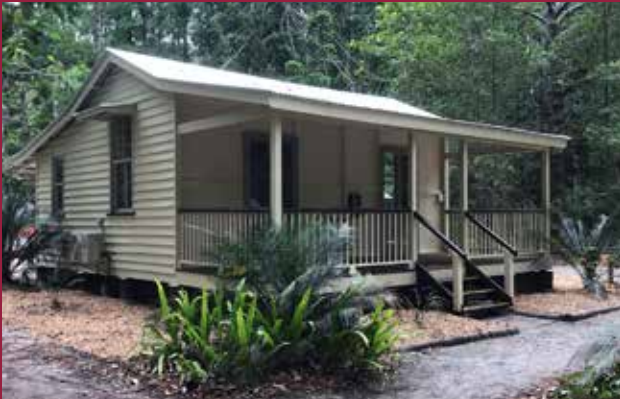
Central Station cottage
