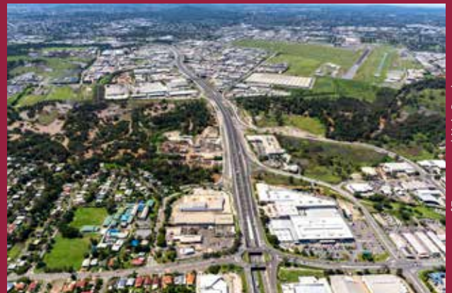
Ipswich Motorway, Rocklea to Darra
