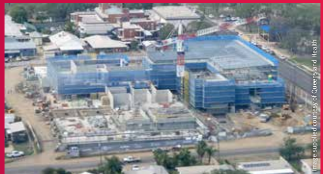
Construction site at Roma Hospital
